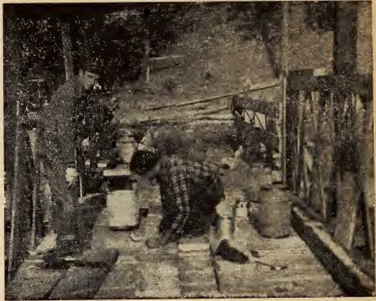
Project work takes up most of the men's time. Here they are shown constructing a bridge across the South Fork of the Flathead River. Other project work includes haying, fence building, telephone line repair, road building and construction of buildings.
